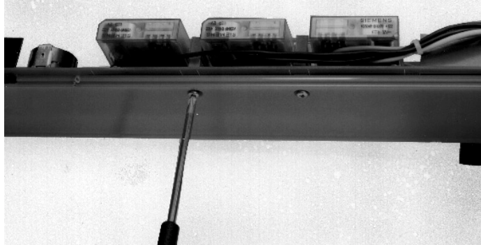
Figure 4-10 Output Relay Replacement
